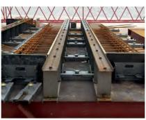
Combination of two Easy Form shutterings with one SPB
